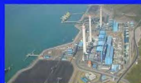
Power Plant Project
